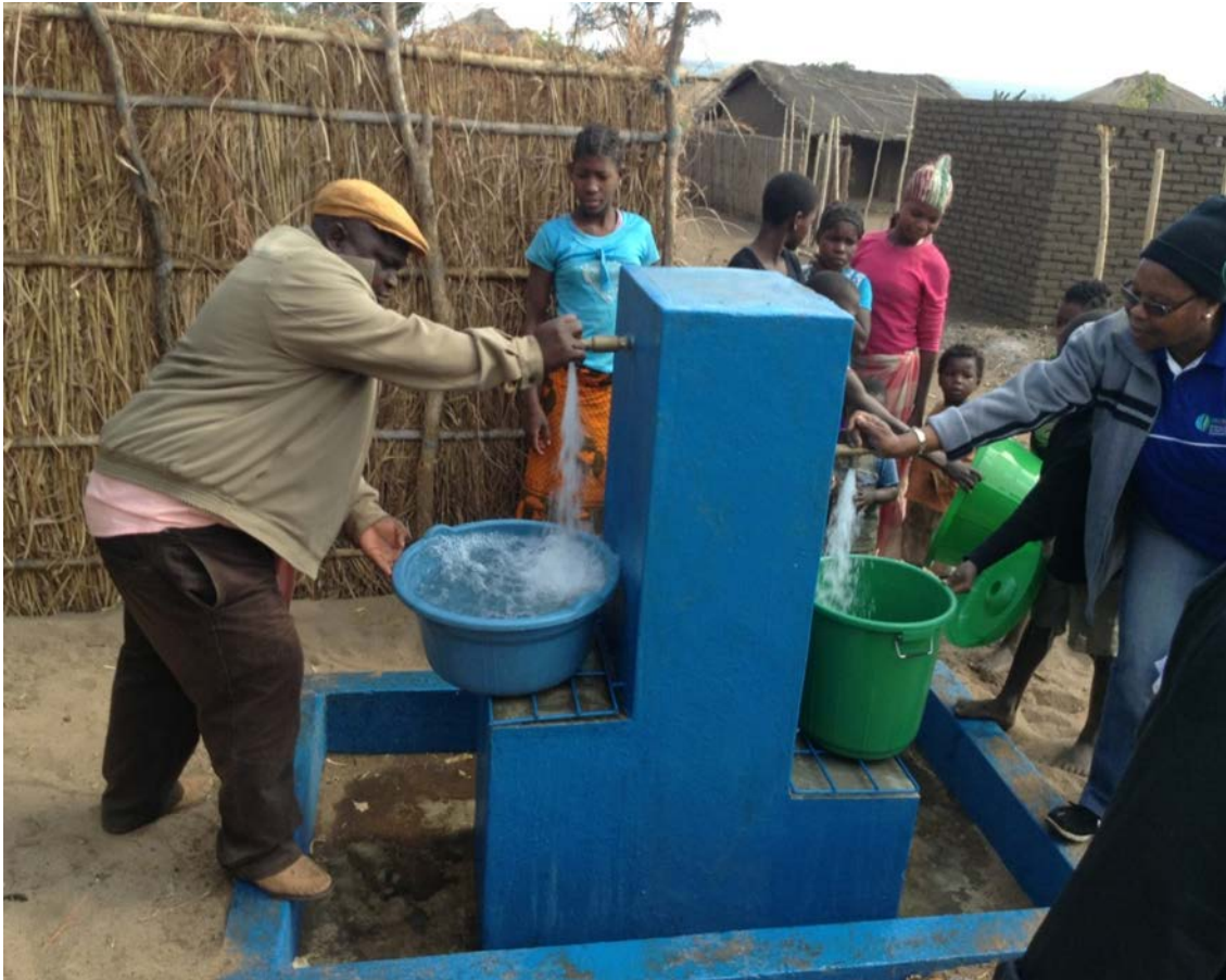
Figure 16. Groundwater source for community in Meponda village, Mozambique [Chaeruca]
