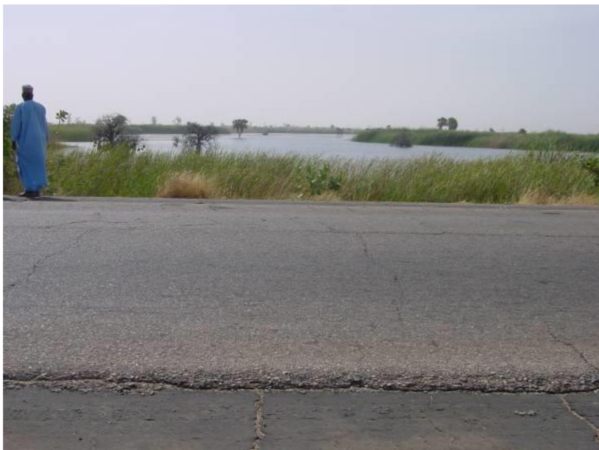
Plate 3: Siltation and Typha Invasion of Ruwan Kanya Reservoir
