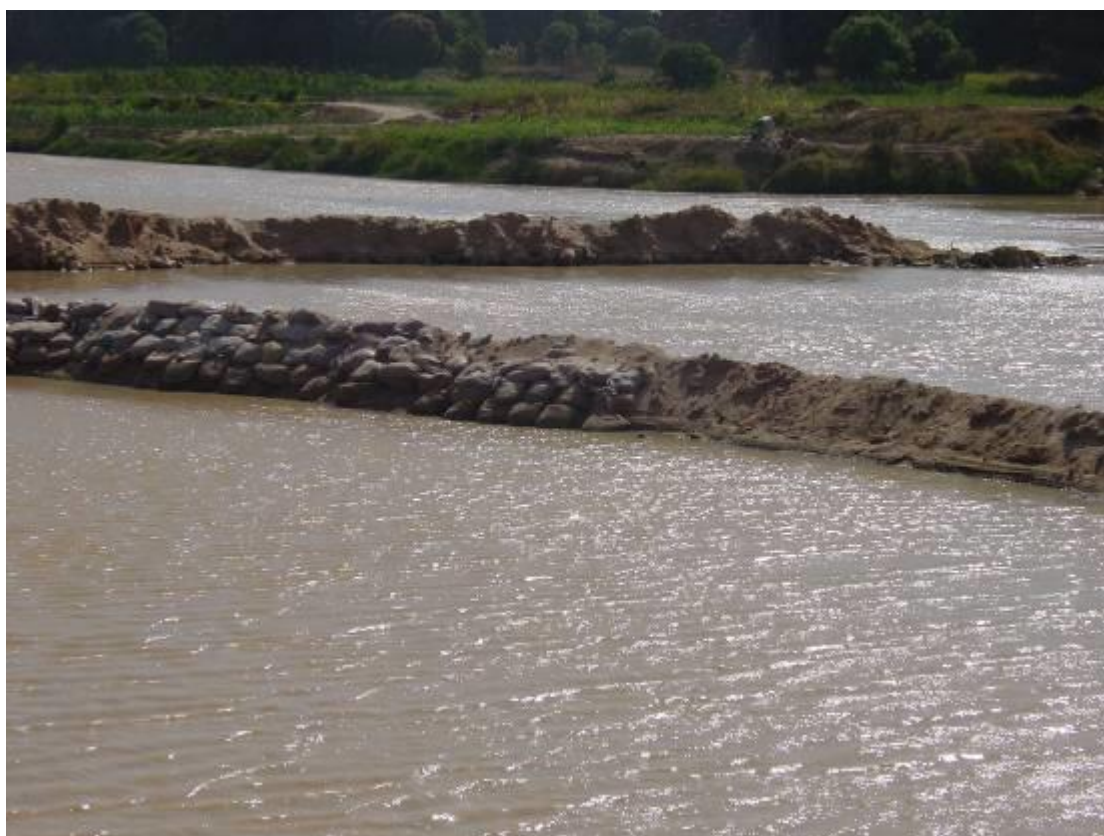
Plate 4: Diversion Structure for KCWS Intake No. 11
